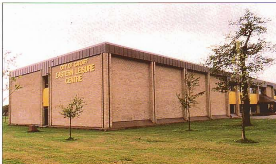
Eastern Leisure Centre, Cardiff
